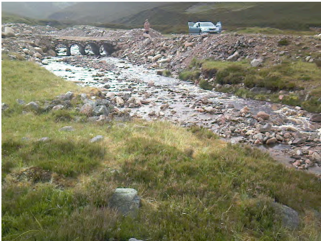
Fig. 2- View looking upstream towards bridge works
