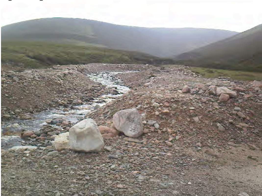
Fig.4- Upstream works/spate debris
